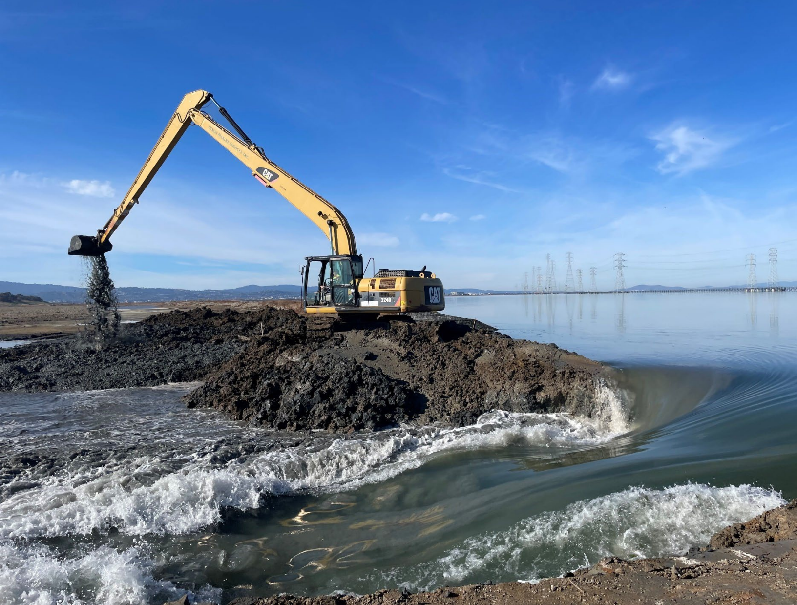
Levee Breach at South Bay Salt Ponds. Photo: South Bay Salt Pond Restoration Project
