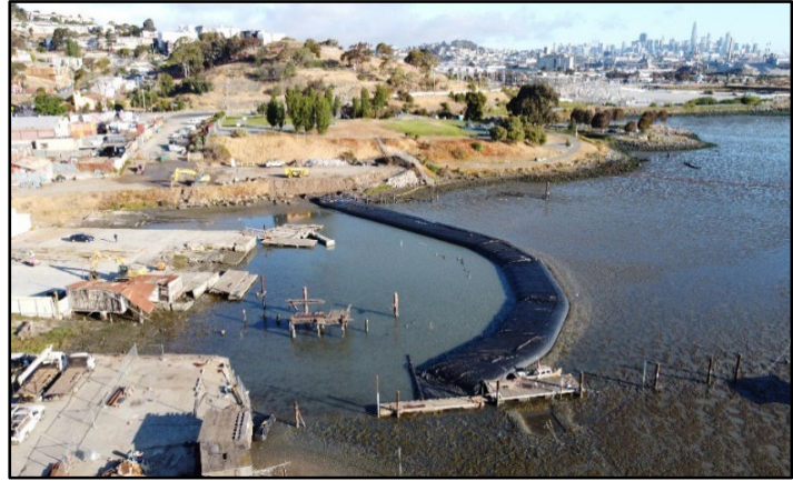
Installed water bladder at 900 Innes Remediation Project
