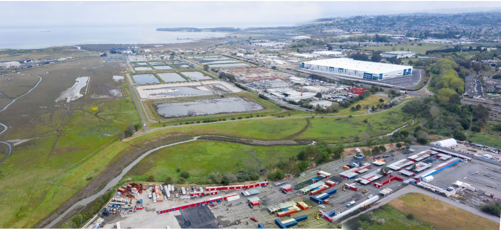
North Richmond Living Levee site
