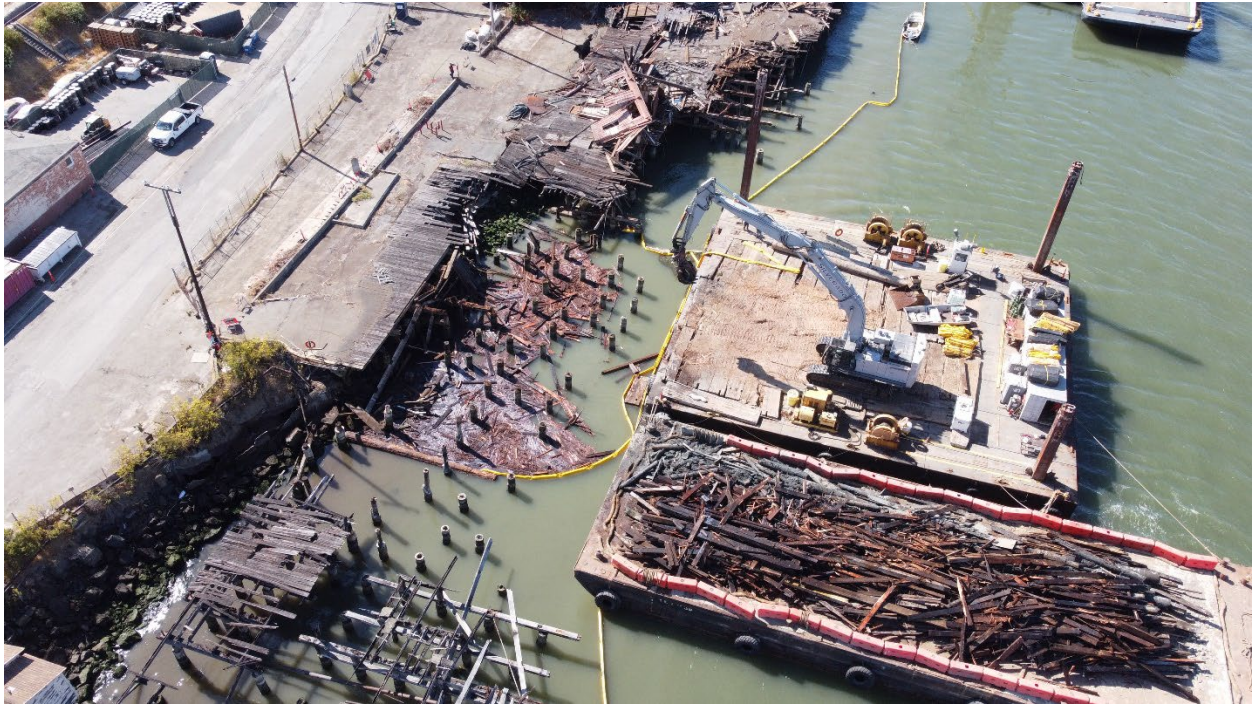
Figure 3. Site cleanup at Terminal 4 Wharf, Warehouse, and Piling Removal Project, Richmond, August, 2023. Imagery credit: Robert Stevens, CSWST2.
