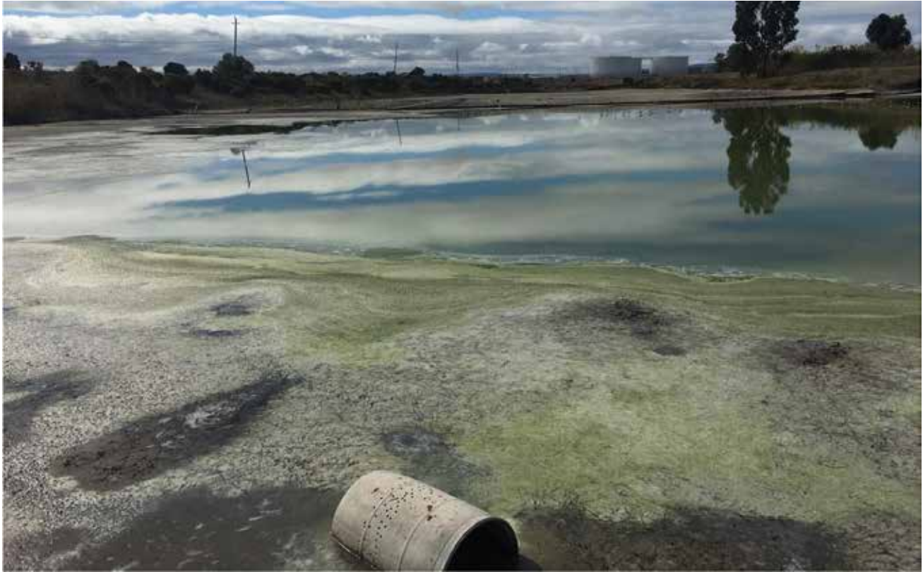
West-facing view of existing storage pond. Portions of the 4.3 acre pond retain water, as shown here. Geotechnical surveys have indicated some contamination, to be addressed with this Project.
