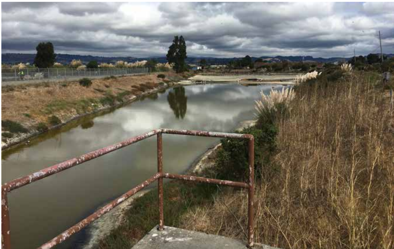
East-facing view of existing storage pond towards San Leandro's WPCP.
