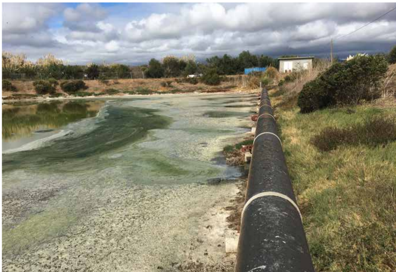
North-facing view of the eastern edge of the storage pond, with an EBDA pipeline that periodically discharges to the pond during peak wet weather flows.
